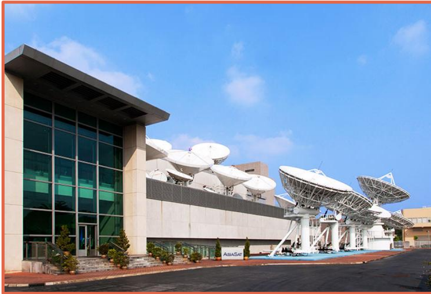
Tai Po Earth Station
